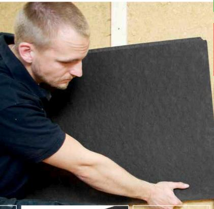
Environmentally friendly insulation materials made from natural wood fibres
